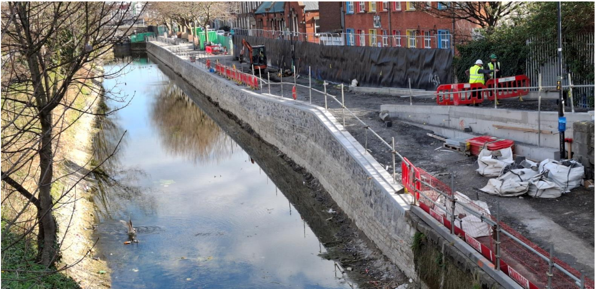
Repaired canal quay wall at Charleville Mall, viewed from Clarke's Bridge
