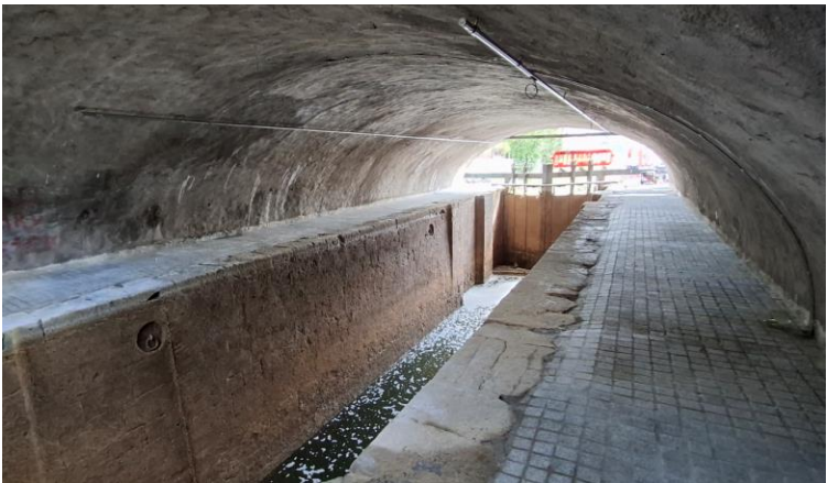
Paving to lock chamber beneath Binns Bridge
